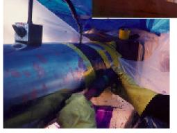
Suspended heated house built around the cylinder enabled crew to work in sub-zero weather. Copper plating was applied to the damaged areas of the cylinder.
